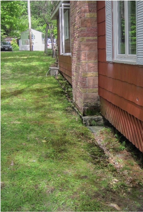
ABOVE LEFT: Runoff from a roof without gutters flows into a dripline. ABOVE RIGHT: An infiltration or dripline trench is a LakeSmart practice that collects and infiltrates runoff, reduces erosion and back splash, and protects the foundation of a structure. Photo credit: Lakes Environmental Association.
