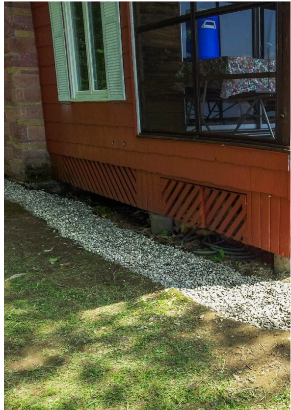
ABOVE LEFT: Runoff from a roof without gutters flows into a dripline. ABOVE RIGHT: An infiltration or dripline trench is a LakeSmart practice that collects and infiltrates runoff, reduces erosion and back splash, and protects the foundation of a structure. Photo credit: Lakes Environmental Association.
