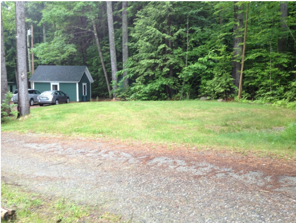
A well-maintained LakeSmart leach field with no smell, seepage, or signs of malfunction Photo credit: Maine Lakes.
