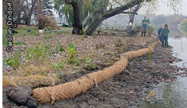
A coir log stabilizes an undercut bank with deep-rooted native species planted above. Source: Minnesota DNR https://www.dnr.state.mn.us/rys/sl/shoreline.html
