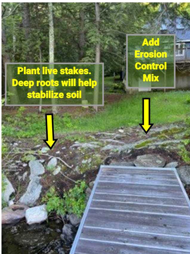
This undercut shoreline is somewhat stabilized by the placement of a log under lip. Planting live stakes on the slope will help with bank stability. Photo credit: Ginger Eliasberg.
