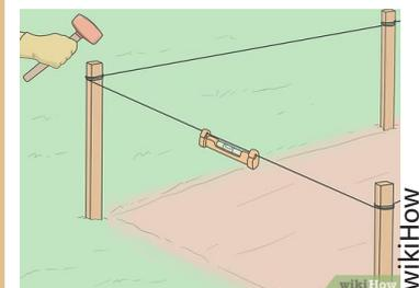
**Measuring slope with string line level.**
