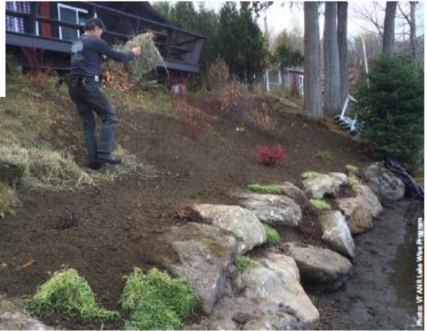
Before (left) and after (right) regrading and installation of a stone toe to protect this bank.
