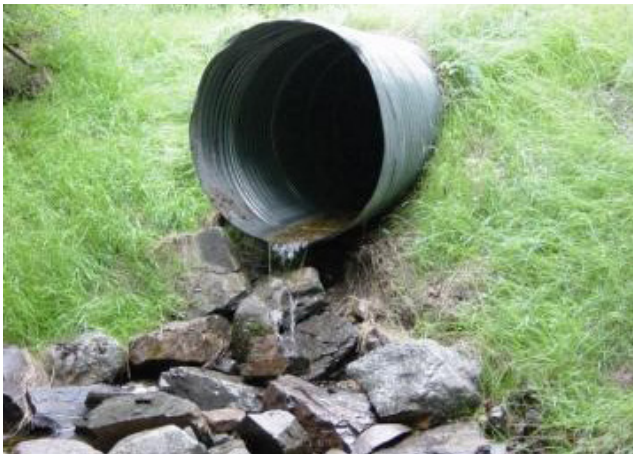
Undersized Culvert
