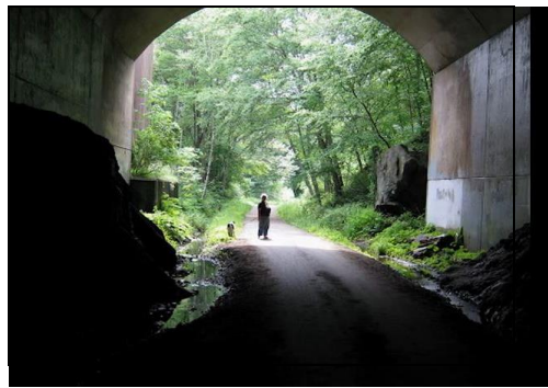
Trail Tunnel at Route 384
