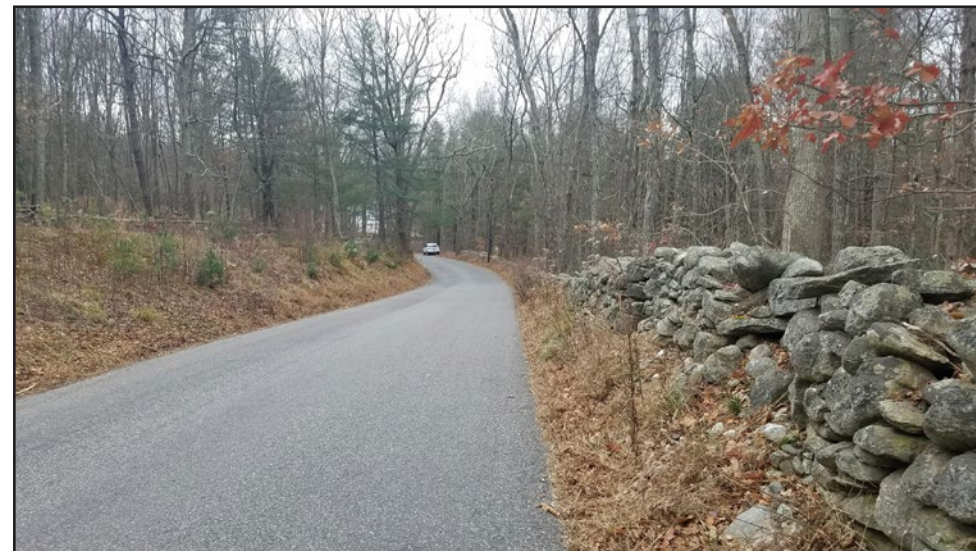
Photo 23 Trail Segment 11 - Parker Bridge Rd. in vicinity of approximate crossing area
