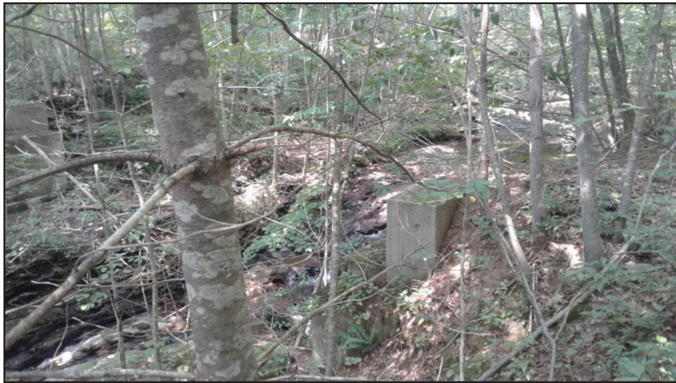
Photo 9 Trail Segment 2 - Concrete abutments on east side of South Rd. at Bolton Pond Brook. Watercourse crossing
