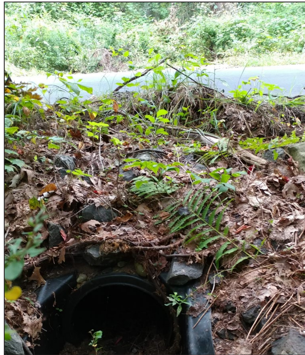
Photo 16 Trail Segment 4 - Culvert beneath Swamp Rd. near approximate crossing area
