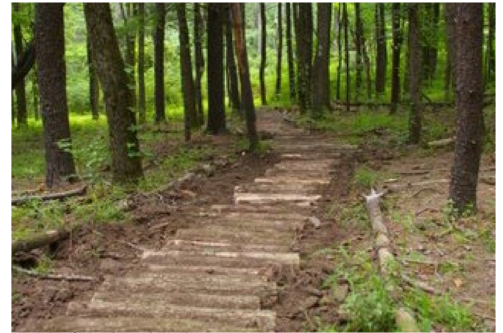
Example of Corduroy through wet area
