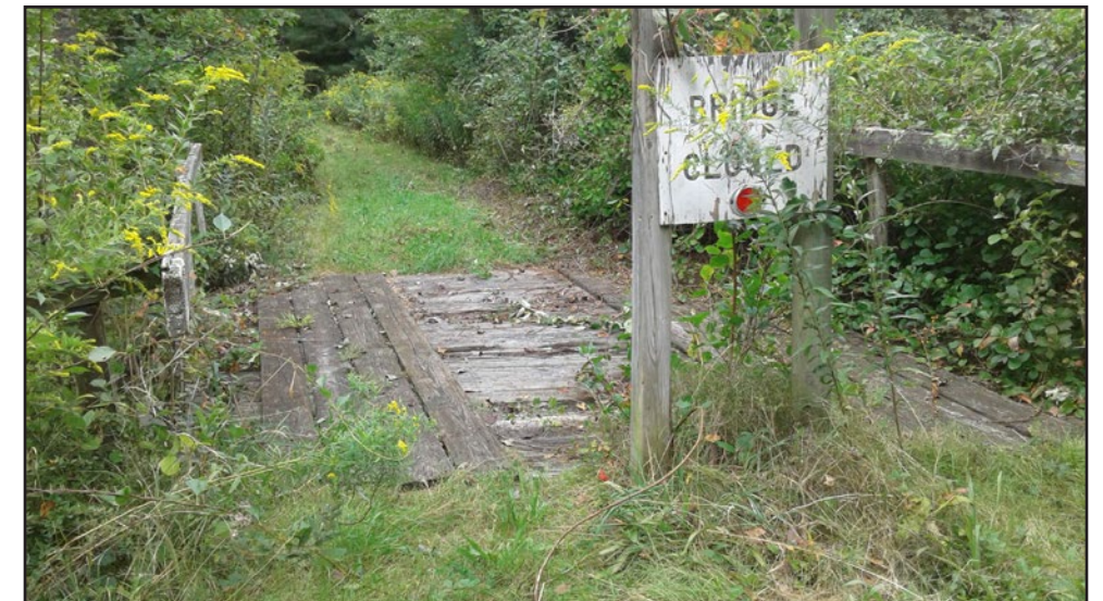
Photo 19 Trail Segment 6 - Deteriorated bridge along potential route on east side of right-of-way to the west of Woodbridge Rd.
