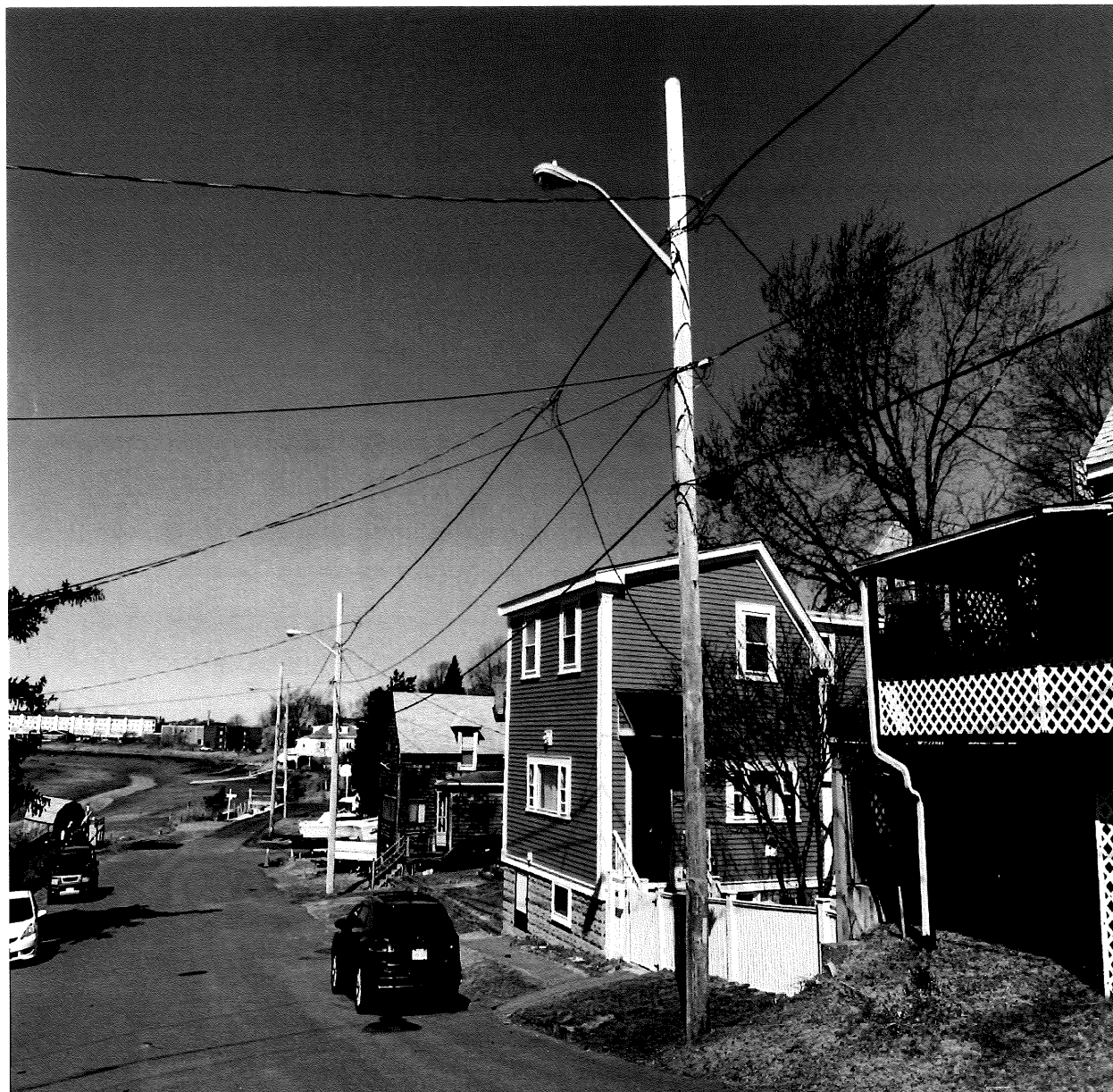
Pole 3090 Located Adjacent to 123 Crystal Ave
