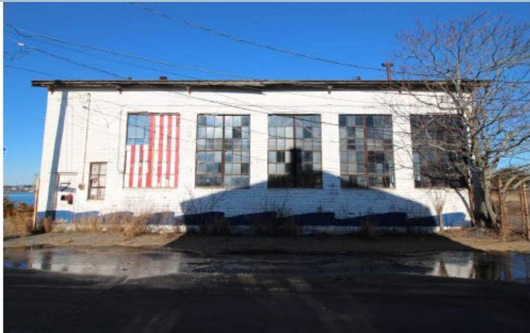
ABOVE view from Thayer Ave
