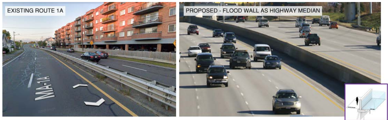
Figure 7-7-6 - Route 1A Flood Wall as Median
