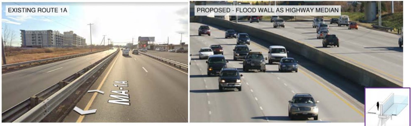
Figure 7-18 - Southern Route 1A Floodwall as Median
