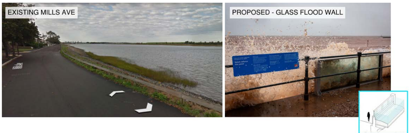
Figure 7-7-4 - Mills Ave Glass Flood Wall
