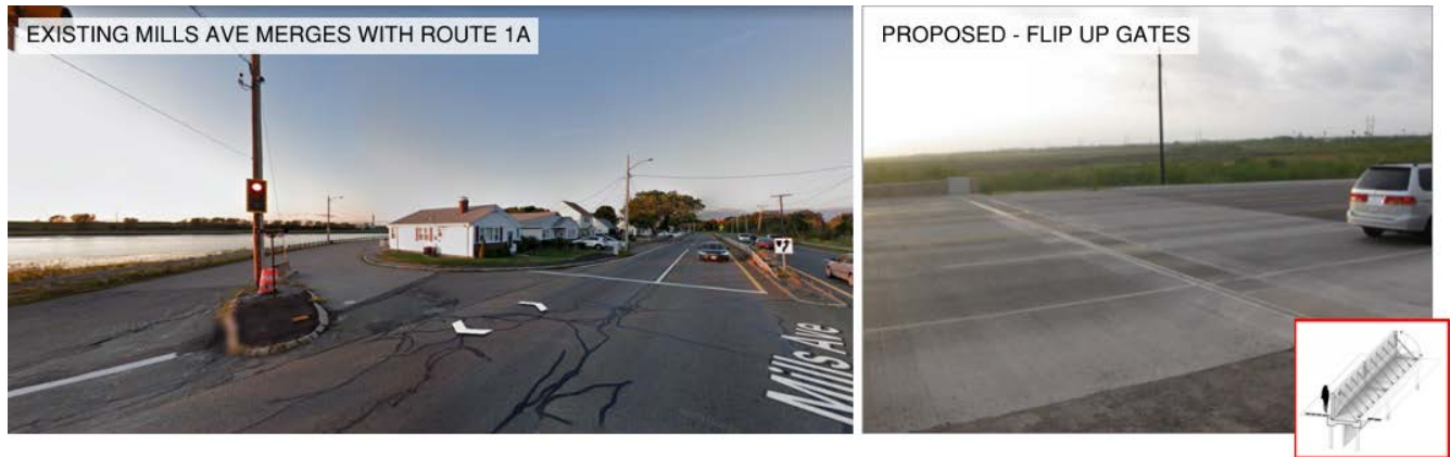
Figure 7-7-5 - Mills Ave Route 1A Intersection Flip Up Gates
