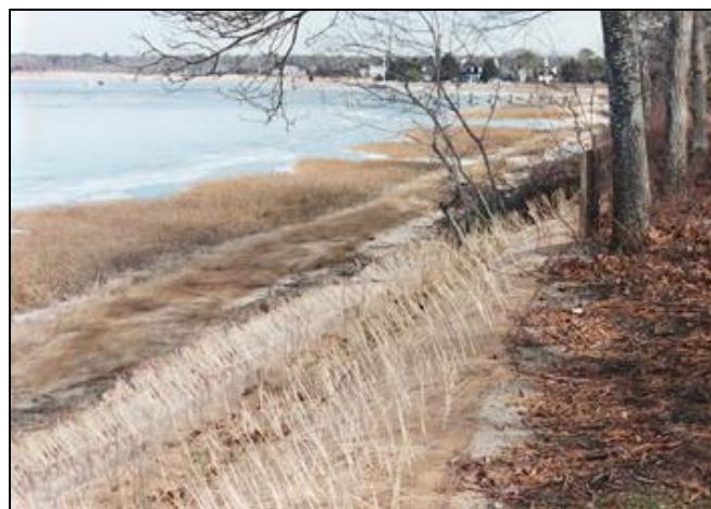
A natural fiber blanket was installed on this bank and vegetation was planted through the blanket while the plants were dormant. (Photo: CZM)
