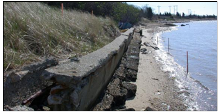
The vertical seawall at this site has been undermined and is failing. In this case, there is room on the site to replace the vertical wall with a sloping rock revetment that does not extend farther seaward onto the beach. (Photo: CZM)
