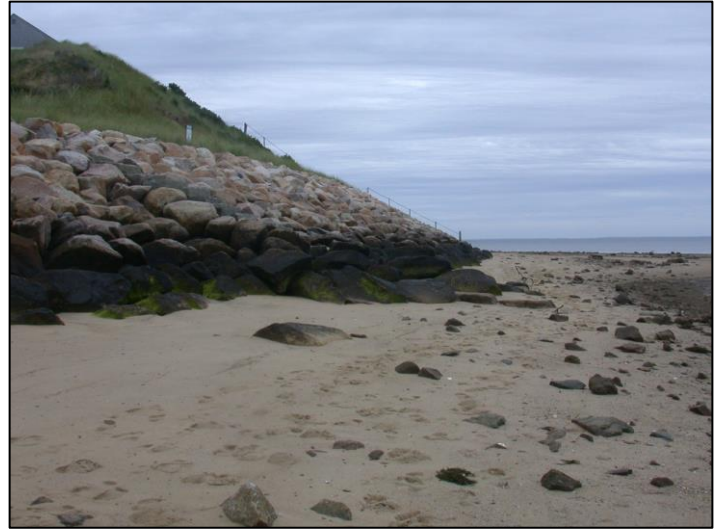
This rock revetment was installed on the lower part of a coastal bank, while salt-tolerant vegetation was planted to protect the upper bank. (Photo: CZM)
