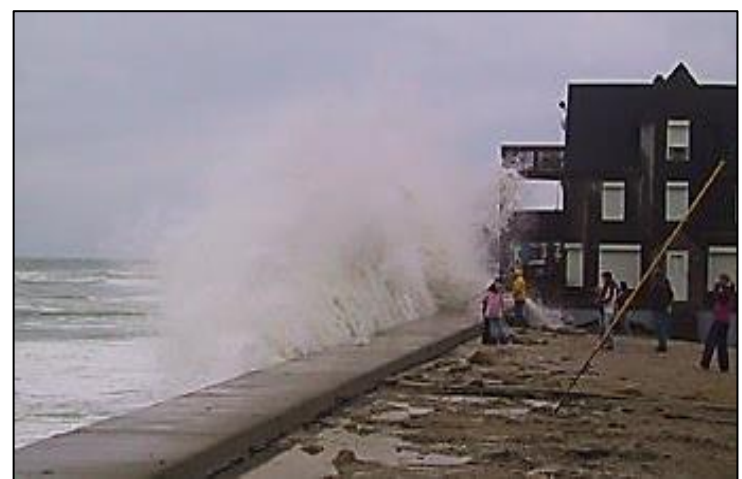
Waves are reflected by this vertical seawall, causing energy to be deflected straight down on the beach and straight up and over the wall, damaging the building behind it. (Photo: CZM)
