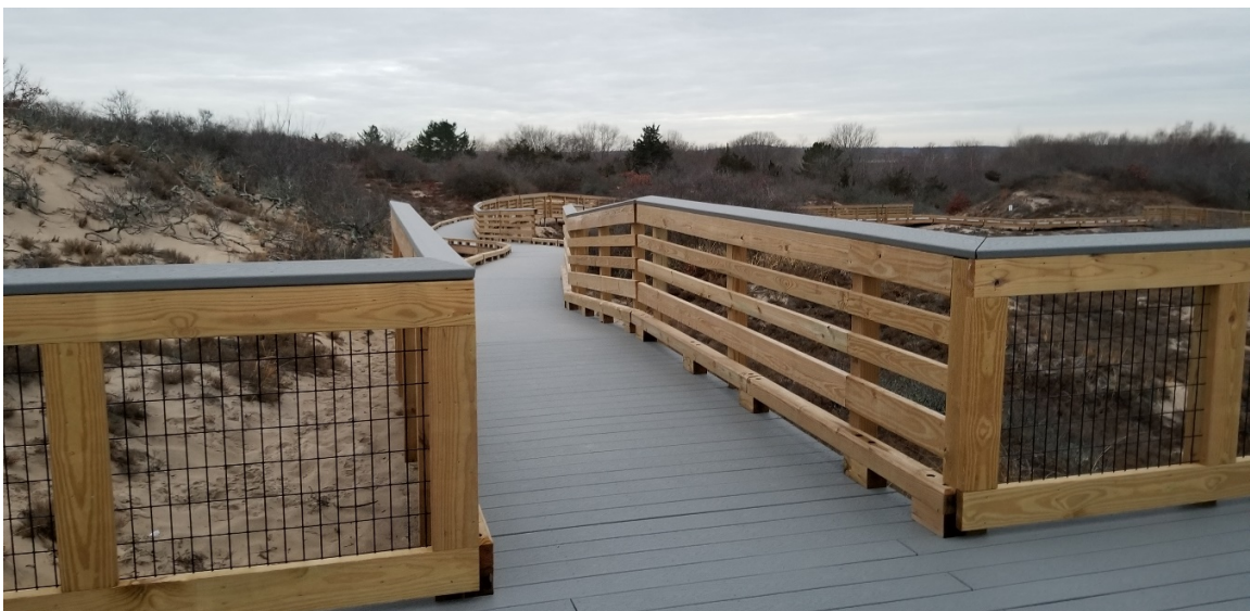
Figure 4. Example of an elevated walkway constructed of a combination of composite decking and wooden framing and handrails (Newburyport, MA).
