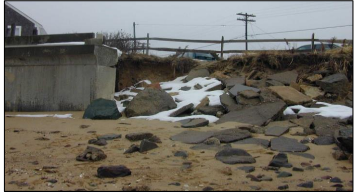
The end effects of this concrete seawall are causing erosion of the bank and damage to the parking area on a neighboring property. (Photo: CZM)
