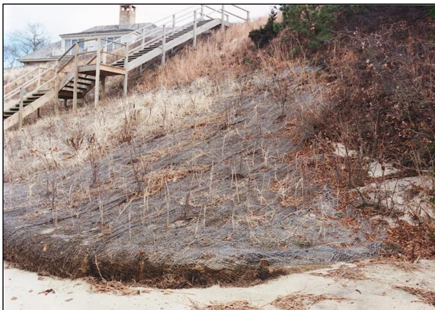
This bioengineering project with coir rolls, natural fiber blankets, and vegetation was designed to minimize erosion on the adjacent property. At the end of the property, the number of rolls was tapered down to one and the bank's slope was reduced and blended in to the adjacent bank. (Photo: CZM)
