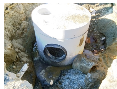
Drainage manhole installation.
