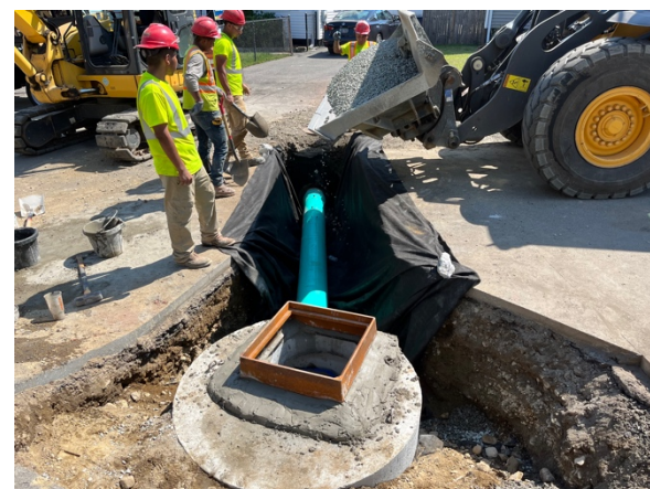
Drainage manhole installation.
