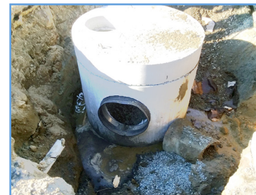
▲ Example of a drainage manhole that will be installed.
