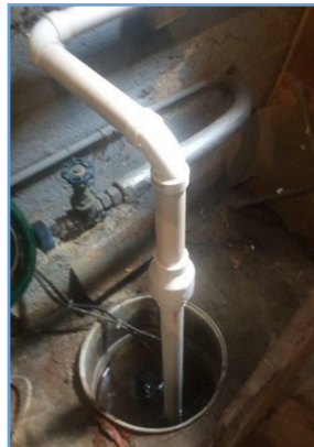
▲ Sump pump ◀ Roof drain
