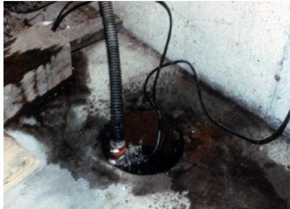
Private inflow from a sump pump
