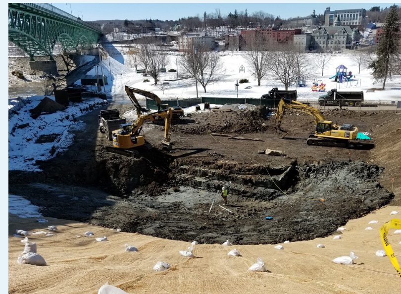
Construction is underway on the third million-gallon wastewater storage tanks GAUD has installed to prevent combined stormwater and wastewater flowing into the Kennebec River.
